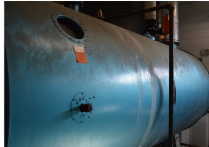
Middle School Original Boilers, Circa 1998 Boiler Condensation
