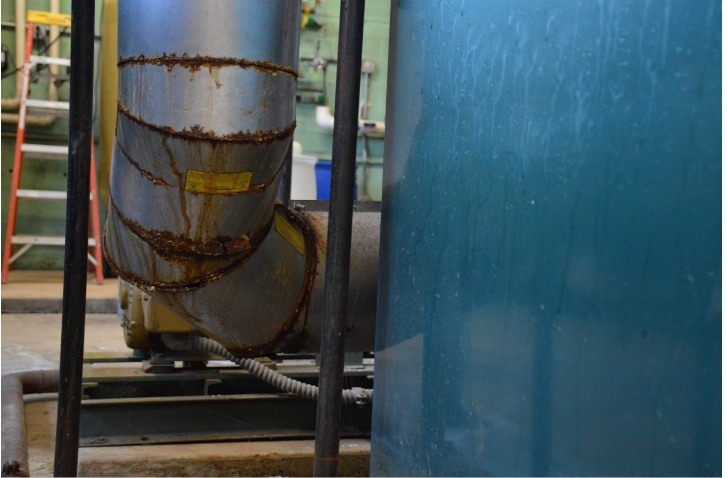
These boilers have exceeded their expected service life [rusty components, corroded pipes.]
