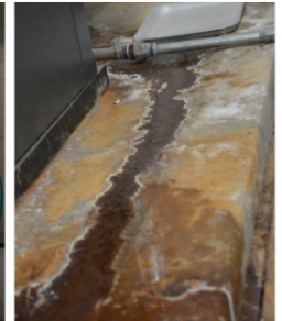
Middle School Original Boilers, Circa 1998 Boiler Condensation
